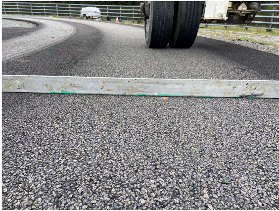
Porous asphalt (P1)
