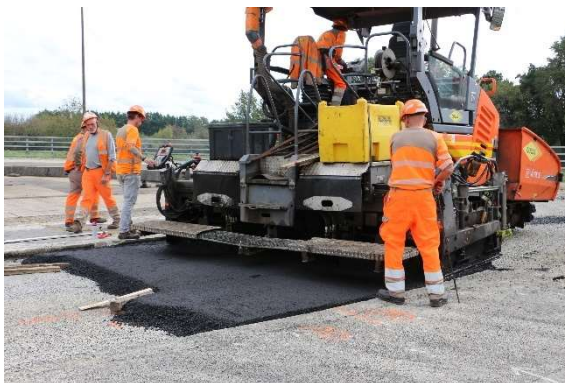
Figure 5. Pictures of GB paving operation
