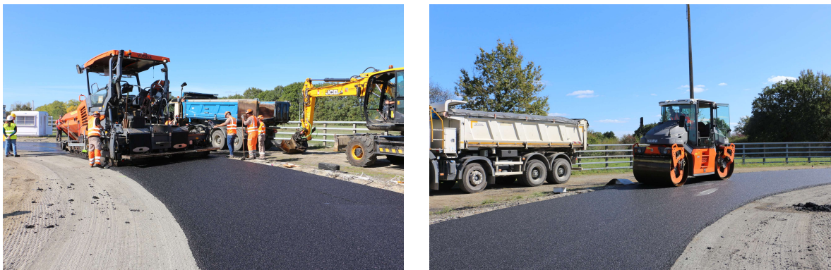
Figure 8. Pictures of paving operation for the Urban section (BB 0/4)
